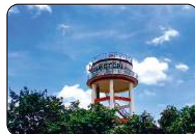
Overhead water tank with sump
