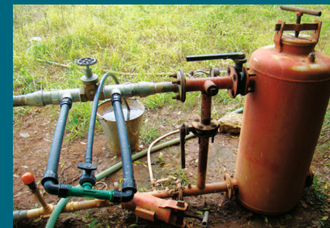
Venturi fertilizer injector system
