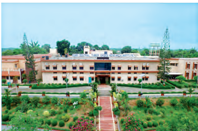
ICAR-CTCRI, Headquarters, Thiruvananthapuram (48.19 ha)
