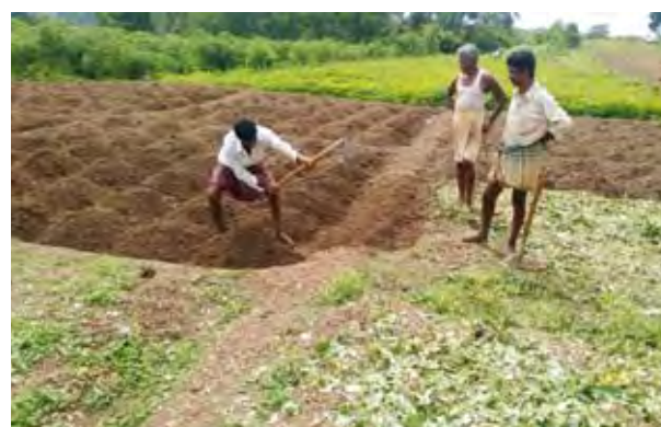
Incorporation and mound preparation
