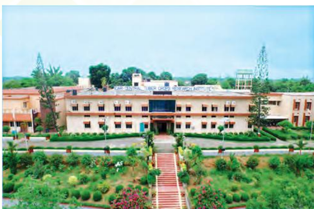
ICAR-CTCRI, Headquarters, Thiruvananthapuram (48.19 ha)
