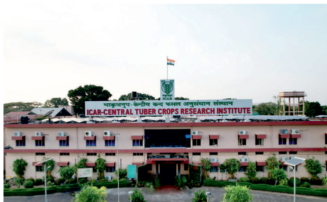
ICAR-CTCRI, Headquarters, Thiruvananthapuram (48.19 ha)
